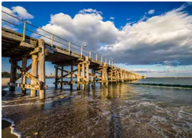
Coffs Harbour Jetty
